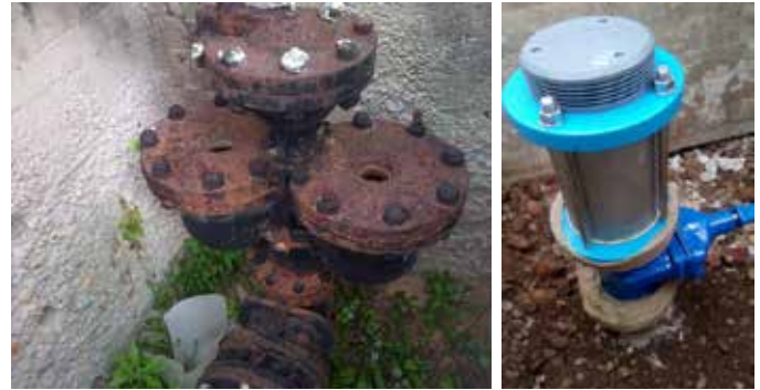
FIGURE 10: Newly replaced air valve
