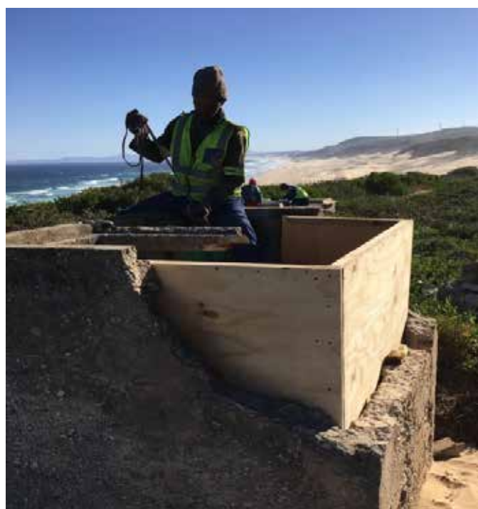
FIGURE 7: Repairing a broken chamber
