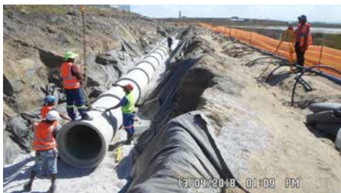
FIGURE 4: Installation of Pipeline (Dry conditions)
