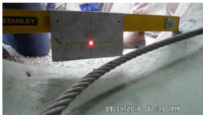
FIGURE 5: Leveling of pipes
