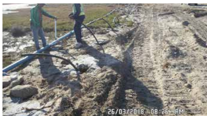
FIGURE 7: De-watering System being Installed
