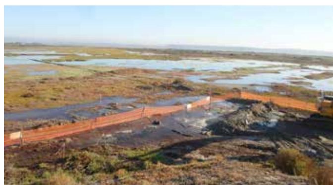
FIGURE 9: Difficult Wet Working Conditions
