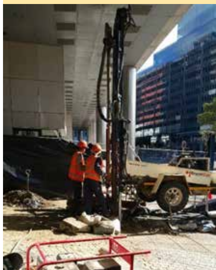
FIGURE 1 (a): Sinking of borehole
